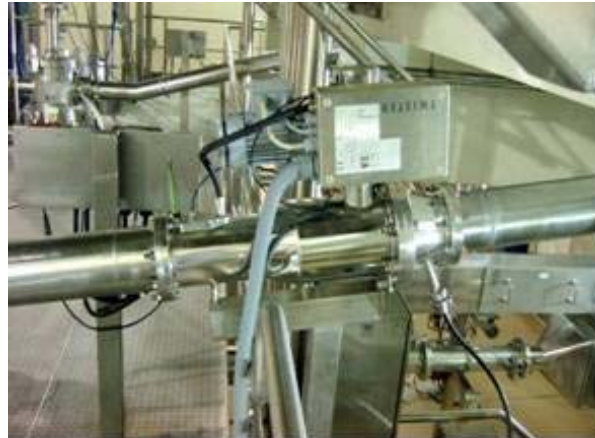
Figure 8: Sampler in 150mm horizontal product line.
